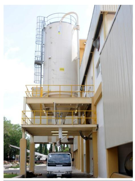
Optimising resource efficiency at Agbara factory Spent grains generated from maize, millet, soya and sorghum during processing at Agbara factory are sent to silo, from where it is discharged to trucks, and sold to farmers for use as livestock feeds.
